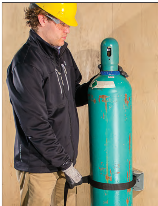
Secure gas cylinders to wall or bench to prevent dangerous tipping.
